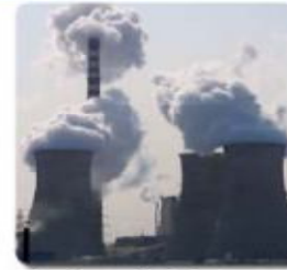
Electric & Gas Utilities
